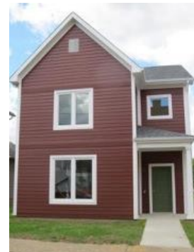
Passive Solar House in Heidelberg
