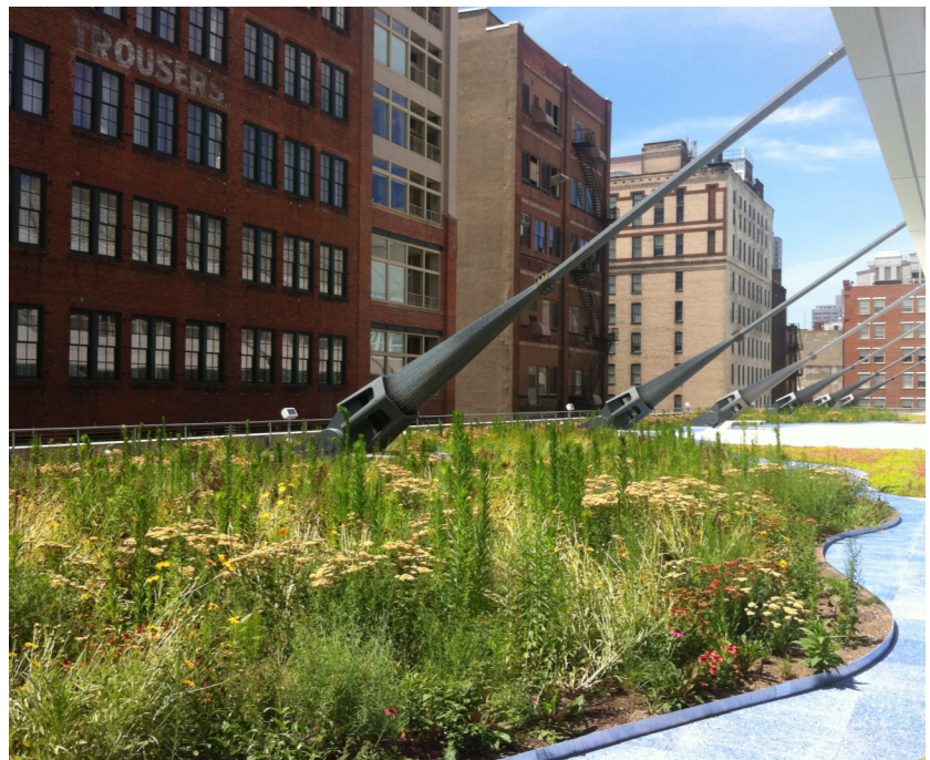
Green Roof at David Lawrence Convention Center
