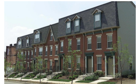
Bedford Hill/HOPE VI development in the Hill District
